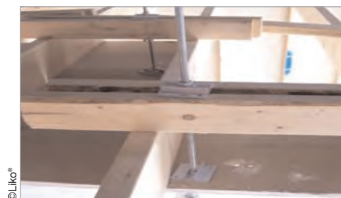
Figure K-11: Threaded Rod Mount
